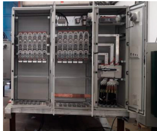
Int. Gral. S5N-6P-2X | 250 a 800 Vac Prot. Fus 200A-800 Vac, 120kA
